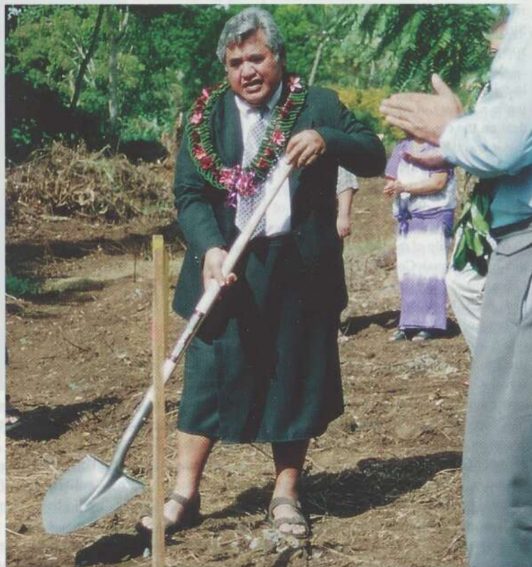
Samoa prime minister Tuilaepa Mallelegaoi turns the soil for the foundation of the multi-million dollar South Pacific Regional Environment Programme (SPREP) headquarters, at Vaillima outside Apia, Samoa
