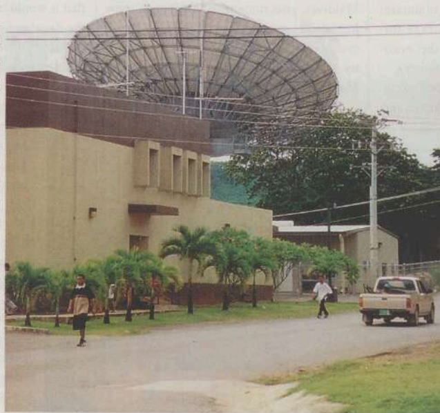
A large satellite dish on the top of the Pohnpei telecommunications building keeps the Federated States of Micronesia in touch with the world
