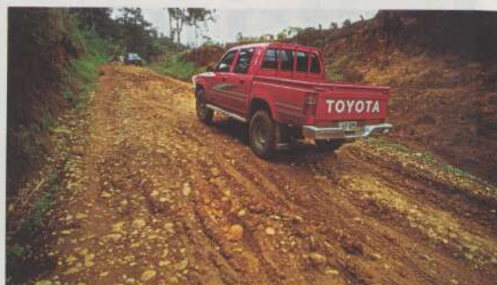
Roads much in need of repair
