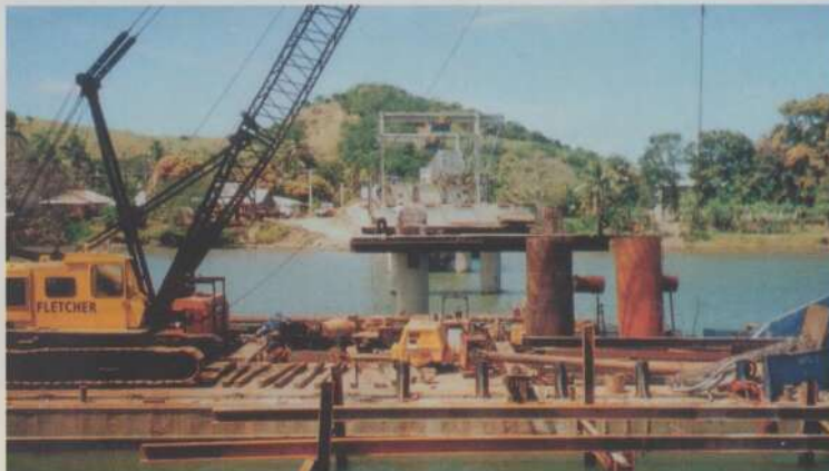
Building bridges ... work in progress on the Sigatoka bridge Picture: Shailendra Kumar
