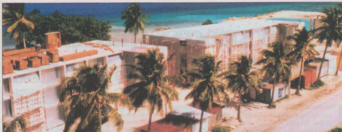
Construction of 150 room Hotel
