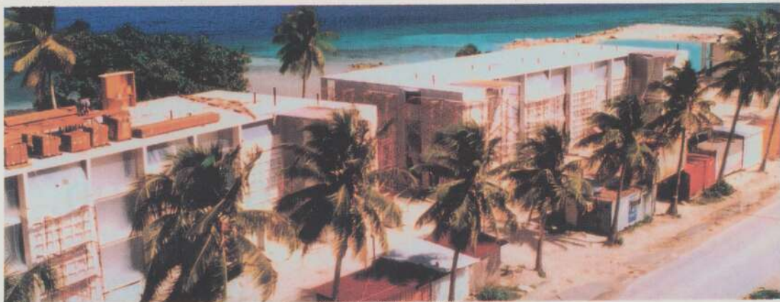
Construction of 150 room Hotel
