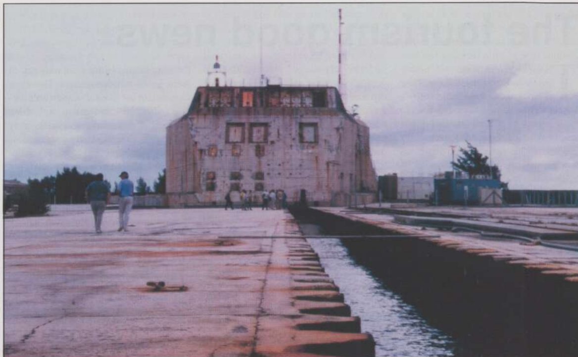
This is Denise, the bunker that housed the control centre during atmospheric nuclear tests at Mururoa. Testing is now done underground and Denise is used for storage. Pictures by ALFRED SASAKO
