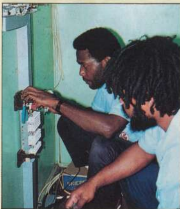
Client service: two linesmen connect telephones for a customer
