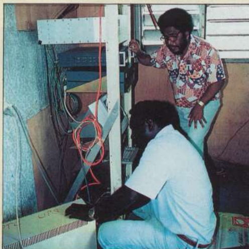
On the job: restoring power supply to domestic satellite equipment in Buin
