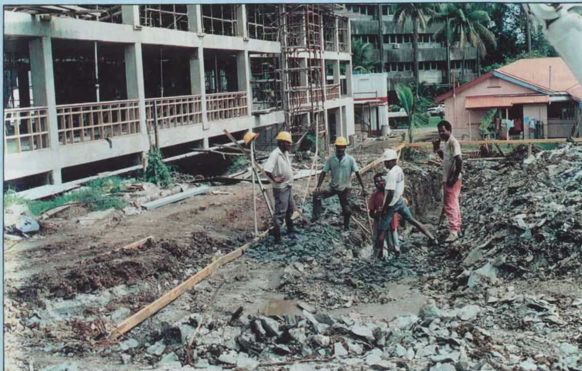
Steady growth: work continues on a Suva construction site
