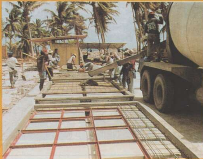
CONSTRUCTION ON A 24 UNIT APARTMENT
