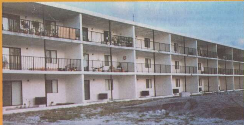
CONSTRUCTION STRUCTURE WAS COMPLETED IN 6 DAYS
