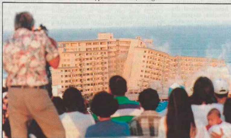
Demolition: the Royal Palm Hotel goes down
