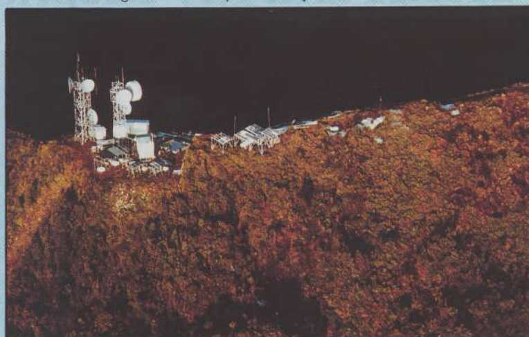
Repeater station: Mt Ialibu Radio Repeater Station, 3410 metres high, is one of the key repeater stations in PNG's telecommunications network
