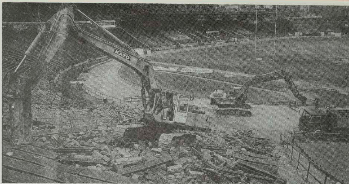
No waiting: With the Sevens rugby tournament over, the demolition of the Hong Kong Stadium gets under way with the removal of seats.
