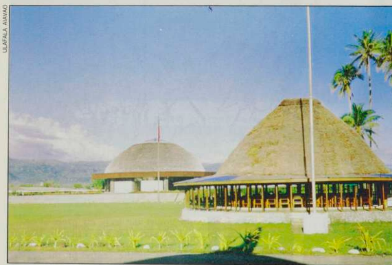
The old and the new: Western Samoa's new Parliament house (background) was closed for repairs and Parliament resumed in the old building (foreground).
