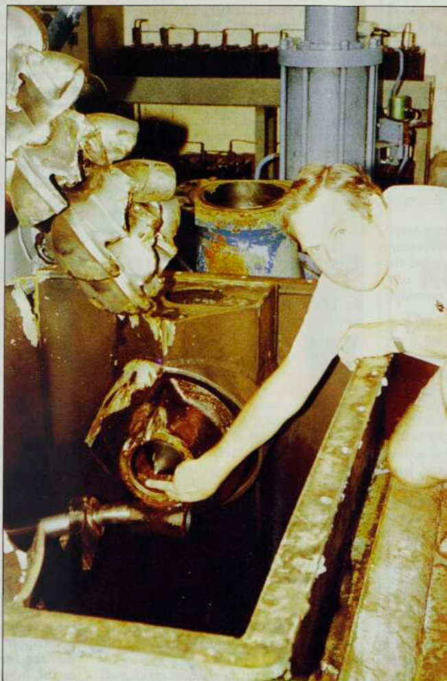
Hussey checks the blocked turbine intake: the hydro generator shook itself to pieces.
