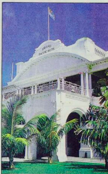
Grand Pacific Hotel: renovation and extension to Five Star.
