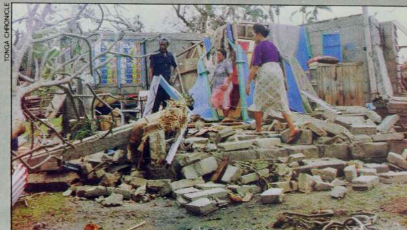
Destruction: two walls remain of this house at Niuaotupapu in the northern Tonga group.
