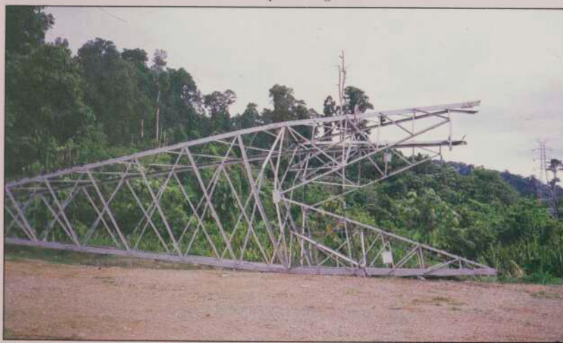
Down: blown power pylon
