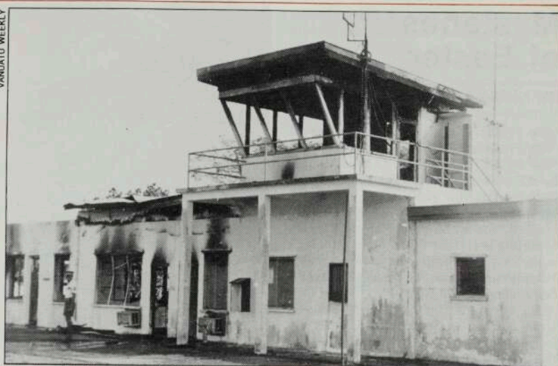
Burnt out: the Bauerfield Airport control tower after the fire.
