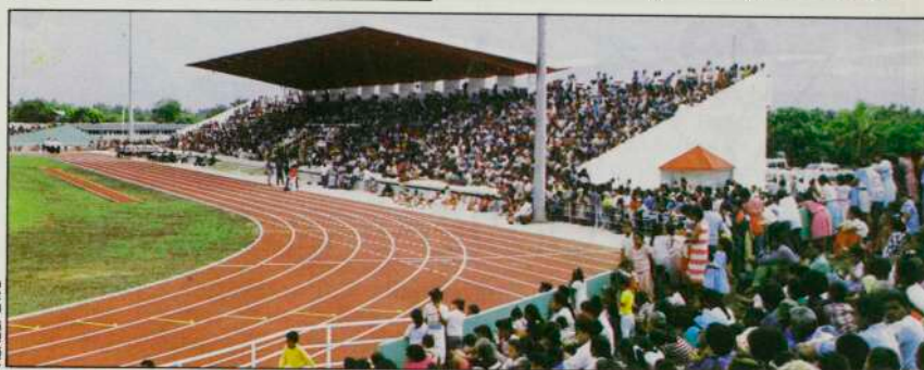
Ready: the new stadium at Teufaiva Park.
