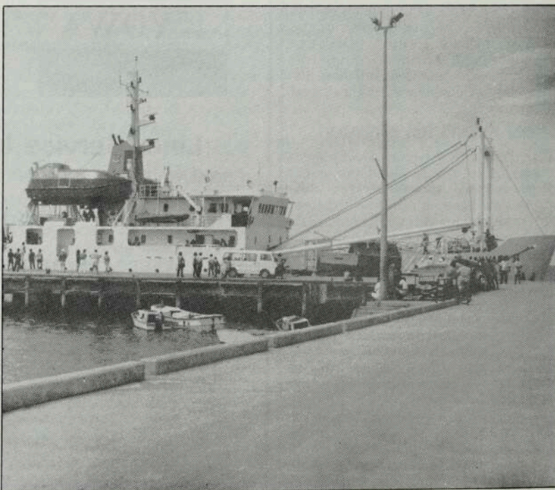
Above: Nivaga II's chief engineer, David Nesbitt, in his gleaming engine room. Right: the new inter-island vessel at her home port, Funafuti.
