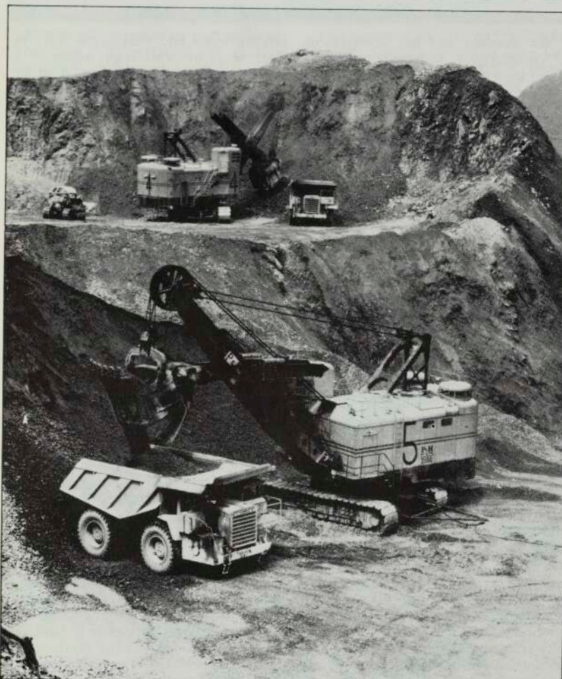
BCL mines around 200,000 tonnes of material per day, using electric shovels. The centre of the dispute is what happens to the 99.52 per cent of rock that does not contain valuable minerals.
