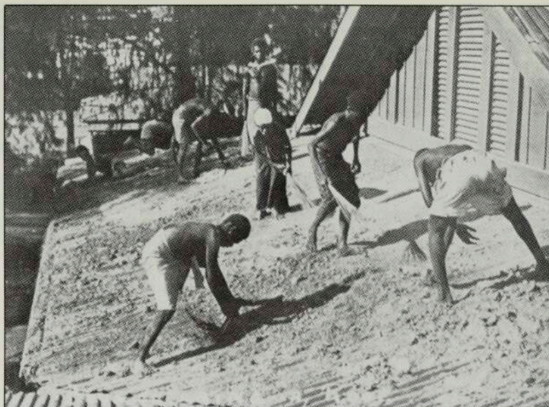
Rain falling on 25-millimetre-deep ash caused roofs and gutters to collapse after the spectacular eruptions of 1937.
