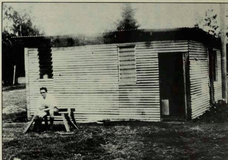
A simple shed was the communications hub of many PNG towns.
