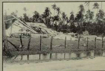
Cyclone damage in the Cooks.
