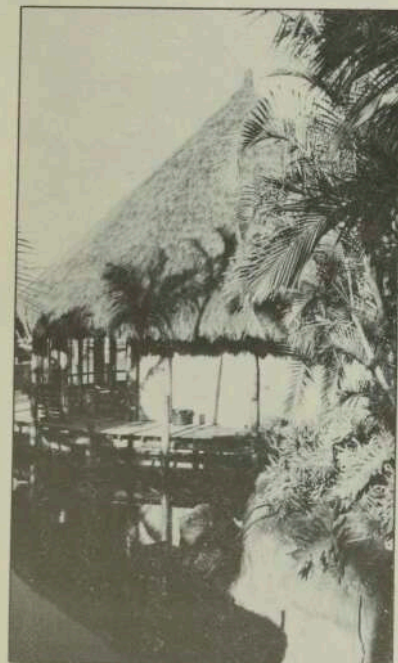
Top: Expo site takes shape. Above: Island lagoon architecture.
