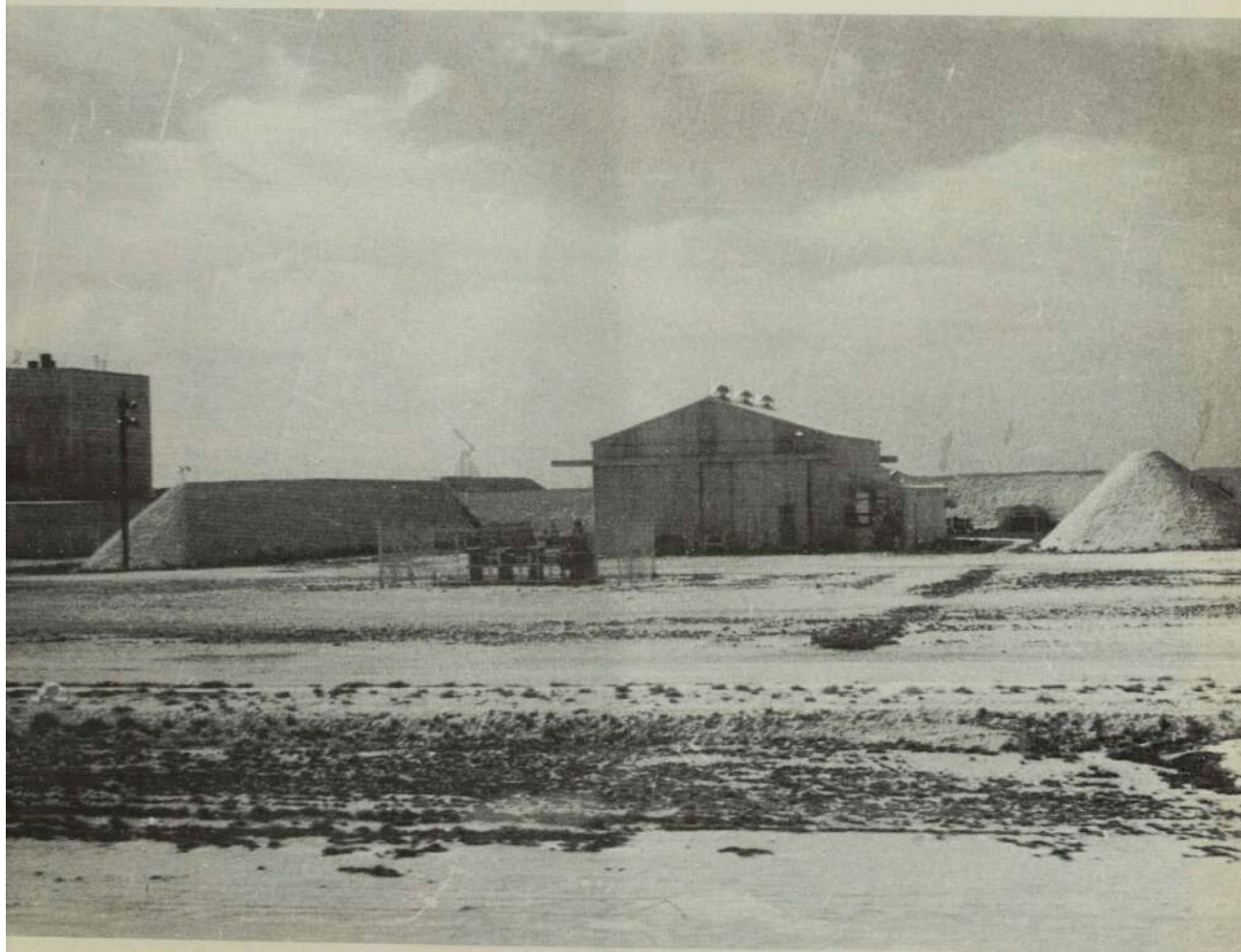
Storage facilities at Johnston.
