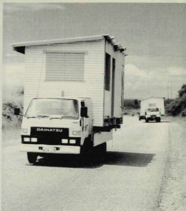
Housing on the move . . . sections of a prefabricated house from J. S. Hill's 'House Factory' in Fiji heads to a site.
