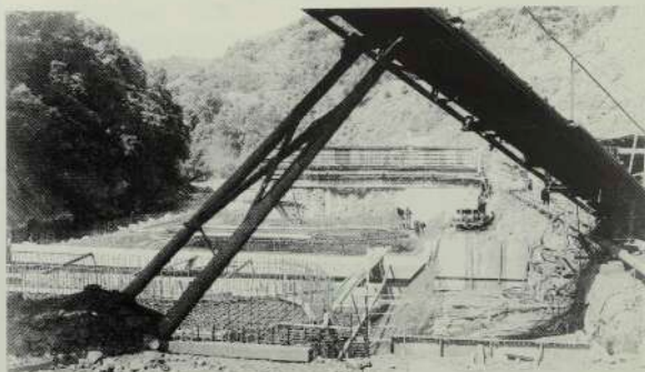
Work on the Monasavu foundations.
