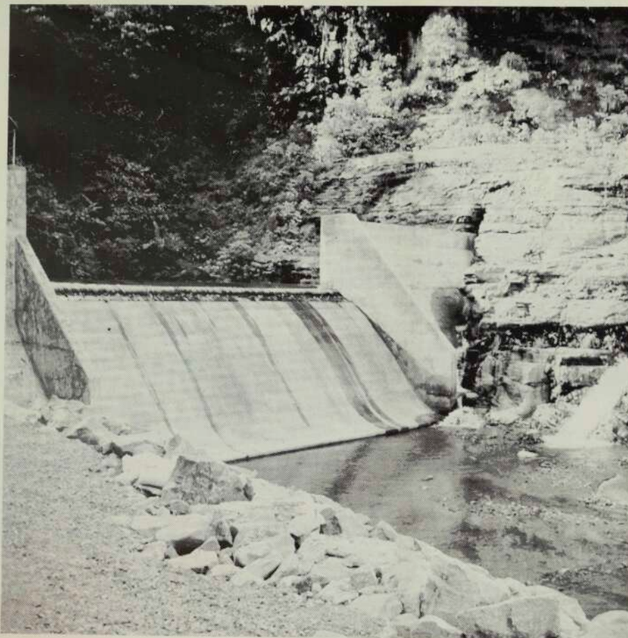
A dam in the giant Monasavu power scheme.
