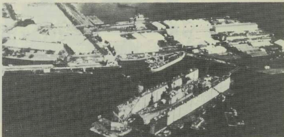
The US Navy's ship repair facility at Subic Bay in the Philippines.
