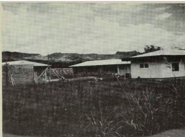
Jail facility under construction at Wamena, Irian Jaya central highlands.
