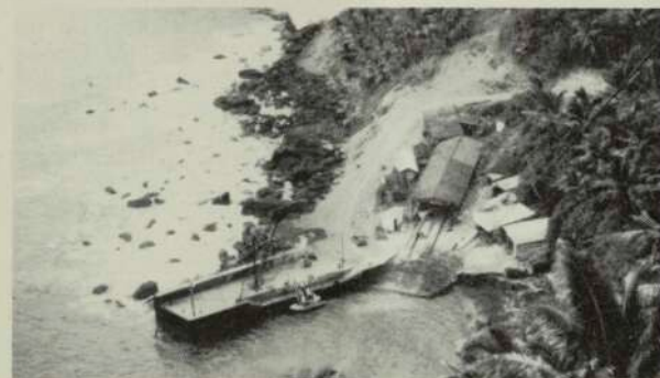
The Pitcairn Island jetty built by the Royal Engineers in 1976. Its square shape caused turbulence in the surrounding water, which eventually undermined it. Above: The remodelled jetty, with its rounded form, has caused the old whirlpool to disappear. Only the half-dozen Pitcairner children are complaining ...
