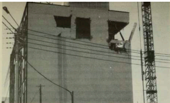
Gaping holes on the top floor of this Noumea building were the offices of Melanesian advancement agencies — before midnight bombers struck. — Sue Williams photo.
