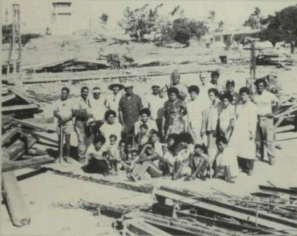
Don Collingwood (fourth from right back row), Managing Director of Sunflower Airlines, with some of the church work crew who demolished the airline's old hangar at Nadi Airport to make way for a new one and to rebuild their church.
