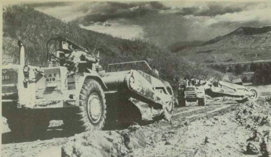
Carving out the future of PNG, these huge scrapers work on cutting roads into the Western Highlands.
