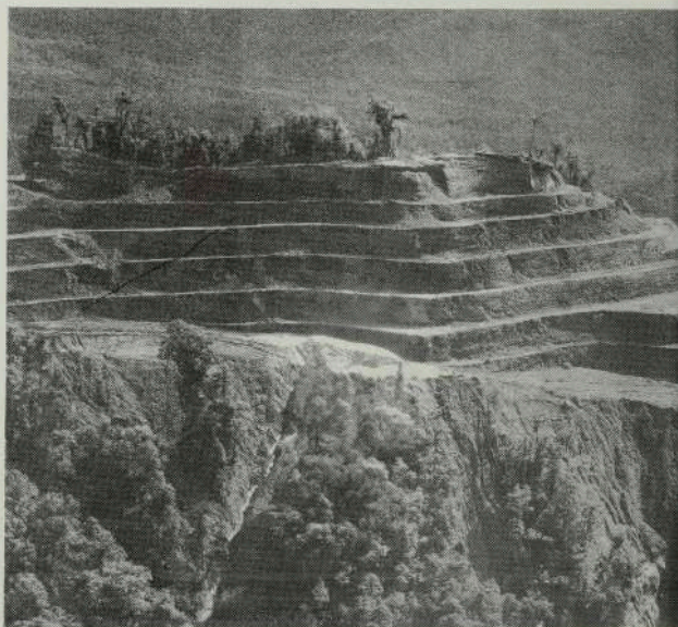
MASSIVE earthworks are a hallmark of the Ok Tedi project . . . like this huge benching on the "Parrot's Beak" outcropping.
