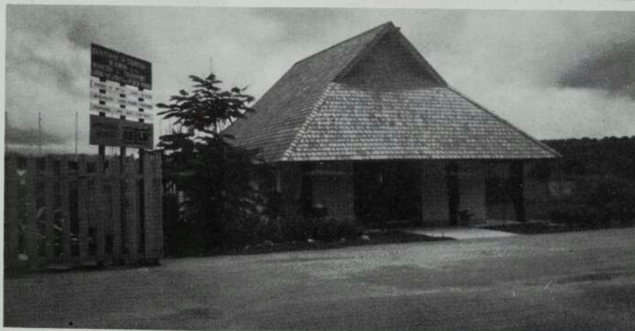
Above: Port-Vila workers on the site of the conference and convention centre which is now a feature of the town's big Intercontinental Hotel. Below: The VIP reception centre at Vila's Bauerfield airport. The Tuesday Sydney-Vila flight introduced this year is becoming known as the "businessmen's" flight due largely to the attractions of the local finance industry.
