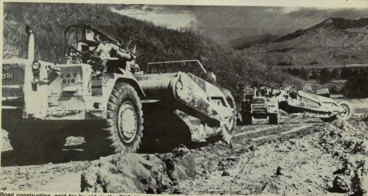
Road construction, paid for by aid, in the PNG Highlands.
