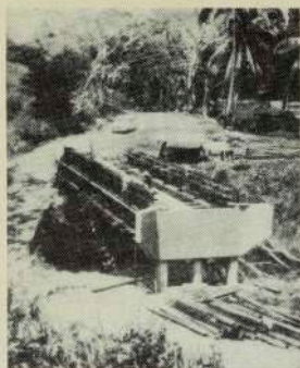
Bridge construction at Gogol, Madang, another aid project.
