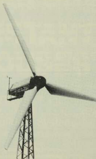
55 KW Wind Turbine
