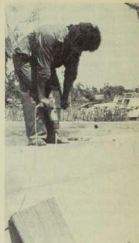
Backed by F.S.P. support a workman repairs water tanks in Haapai after Cyclone Isaac.
