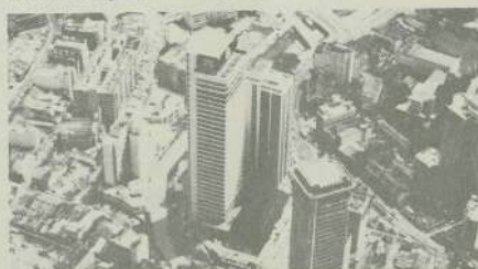
Menara Bumiputra, the Bank's HQ in Kuala Lumpur, Malaysia.
