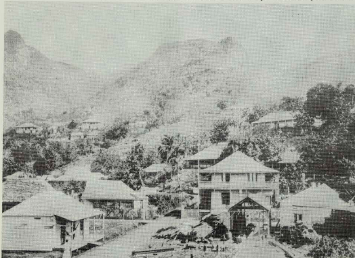
Old Levuka ... how many of these buildings have been preserved?
