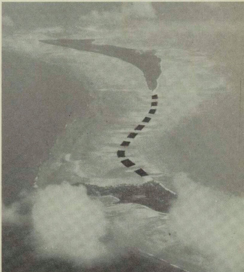
Dotted line shows position of projected causeway between Bairiki (lower) and Betio islets, Tarawa, Gilbert Islands. — Picture by courtesy RNZAF.
