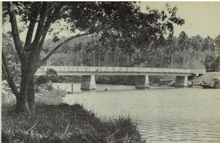
Once more the Renee River near Santo in the New Hebrides can be crossed in comfort and in safety via this new bridge which was opened with a ribbon-cutting ceremony, by the wives of the British and French district agents, Mrs Turner and Mrs Valentini. Built by the Citra Construction Company of Noumea in New Caledonia and designed by Wilton and Bell, Dobbie and Partners, consulting engineers, of Sydney, the bridge replaces a badly battered, low-level concrete bridge at which nature had two attempts at destruction. It was badly damaged and closed to traffic as a result of the November, 1971, earthquake and then washed away by floods created by cyclone Wendy in 1972. A ferry service has functioned for nearly a year. Wilton and Bell, Dobbie and Partners were consulting engineers for the new Vila wharf.
