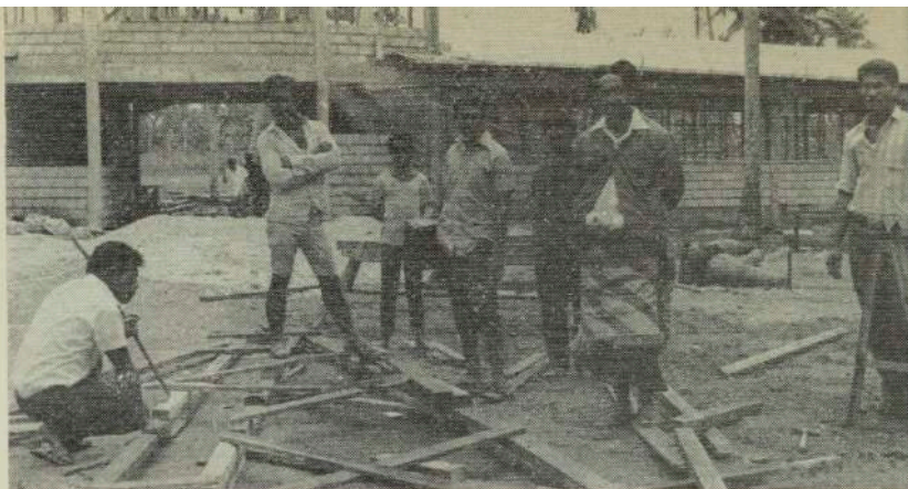
Futa supervises the building of his new Athens.—Photo: Inese Civkulis.
