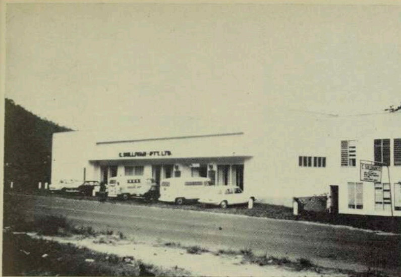
The new warehouse and offices at Rabaul.
