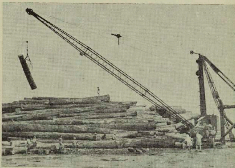
An electric crane at Lever's Pacific Timbers, Kolombangara, lifts logs from a truck (right) for workers to cut, measure and mark and then place on the stockpile.
