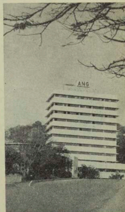
Things are different today. The recently-opened, 12-storey ANG House now dominates Port Moresby's skyline.
