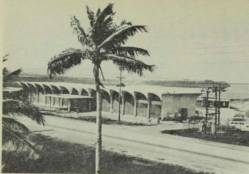
● Guam's new SEACOM cable station
