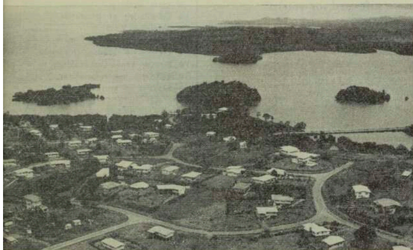
This is a partial view of the Bay of Islands, where a new hotel is being built. The hotel site is further round to the right.—Photo: Stinsons.
