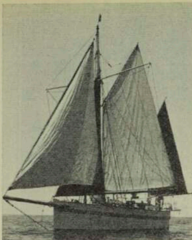
"Lucent" under sail. The large yard arms are part of an efficient self-steering system, which operates with winds from any quarter.
