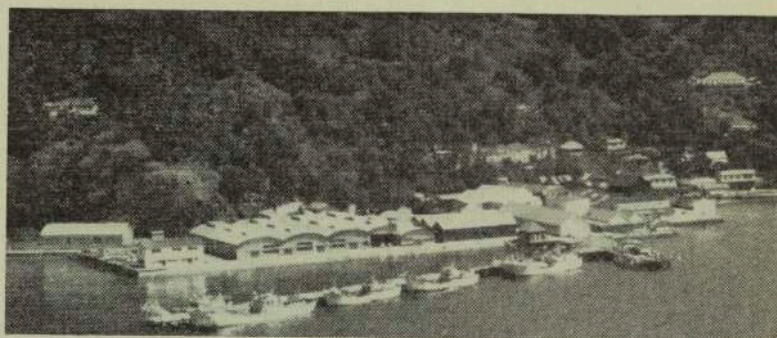
Levuka's present fish-freezing factory was opened in 1964. It is seen in this aerial picture with five Japanese fishing boats alongside the wharf.
