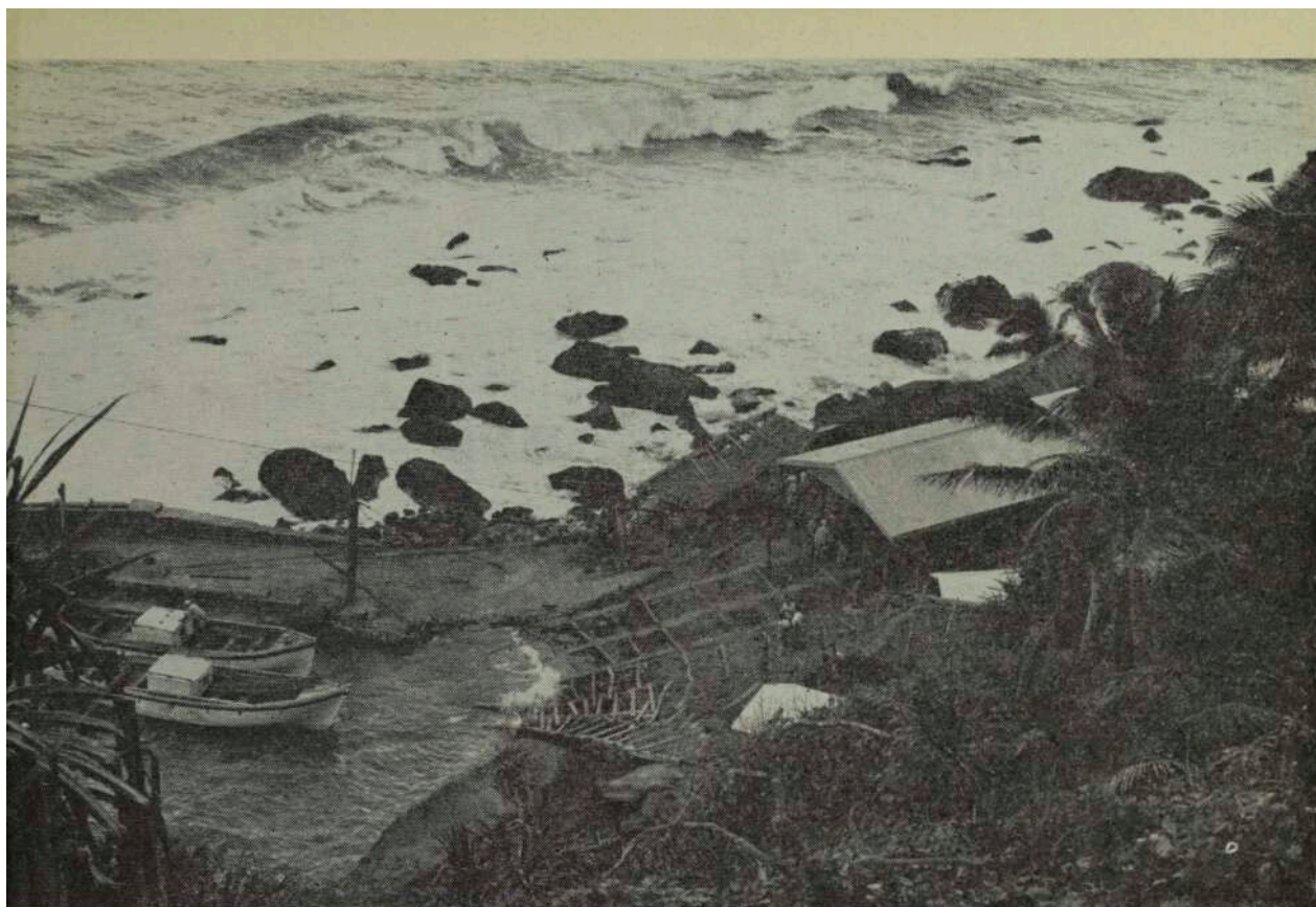
An extension of the jetty to give greater protection to the tiny basin, and the erection of a better boat-house and slipway, have at last brought changes to Pitcairn's famous Bounty Bay.
