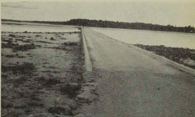
The Andersen Causeway from the Bairiki end. This and another similar structure give Tarawa 20 miles of motor road along the southern chain of islets.
