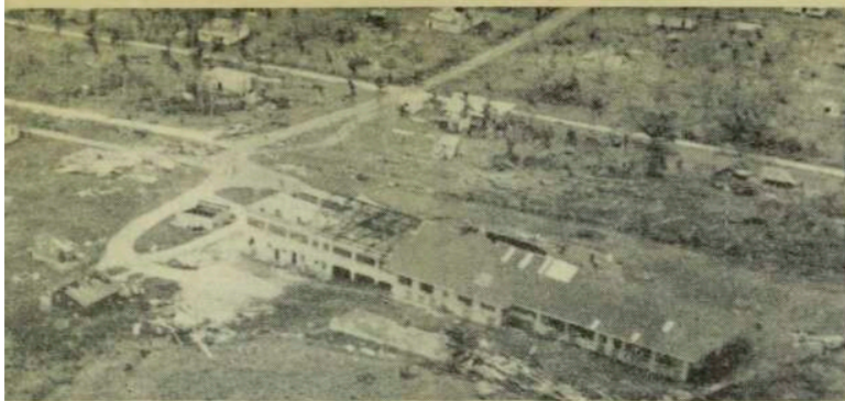
These aerial photographs of Vavau show some of the damage of the Tongan hurricane. At top, is the big concrete hospital at Neiafu, partly unroofed, and below, the scene of desolation nearby. Photos: S. A. Whippy
